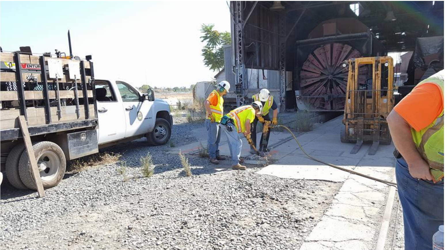
Jack-hammering begins on the north Firing Line track
