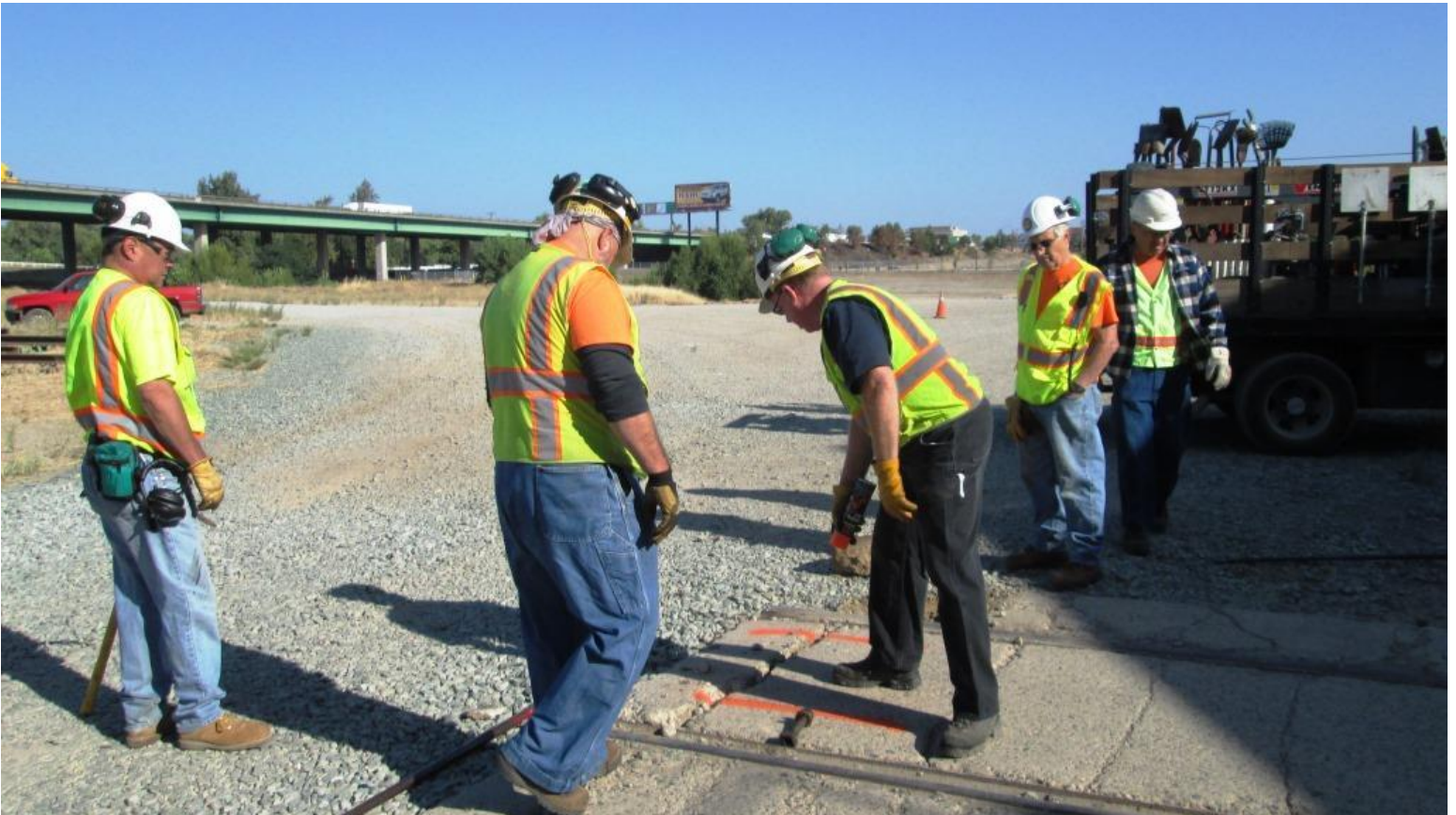
"H" marks the spot – or something like that. Ed M. marks the area of concrete to break-up
