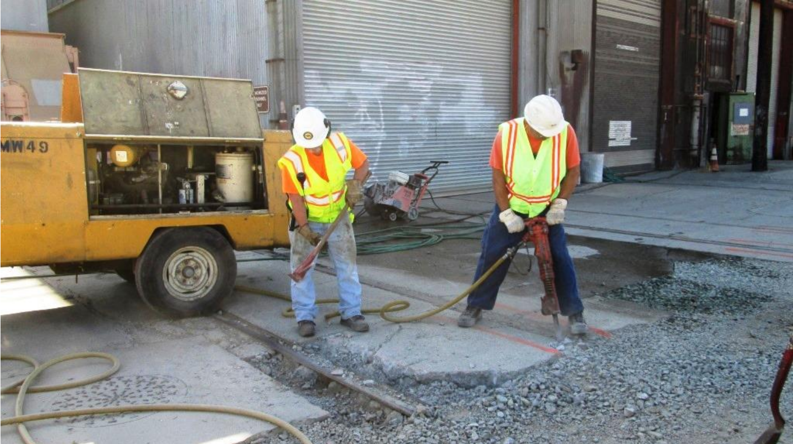
Second shift: Joe clears away rubble as John jack-hammers
