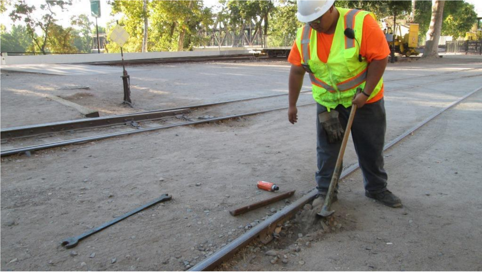
Anthony digs-out the offending joint-bar
