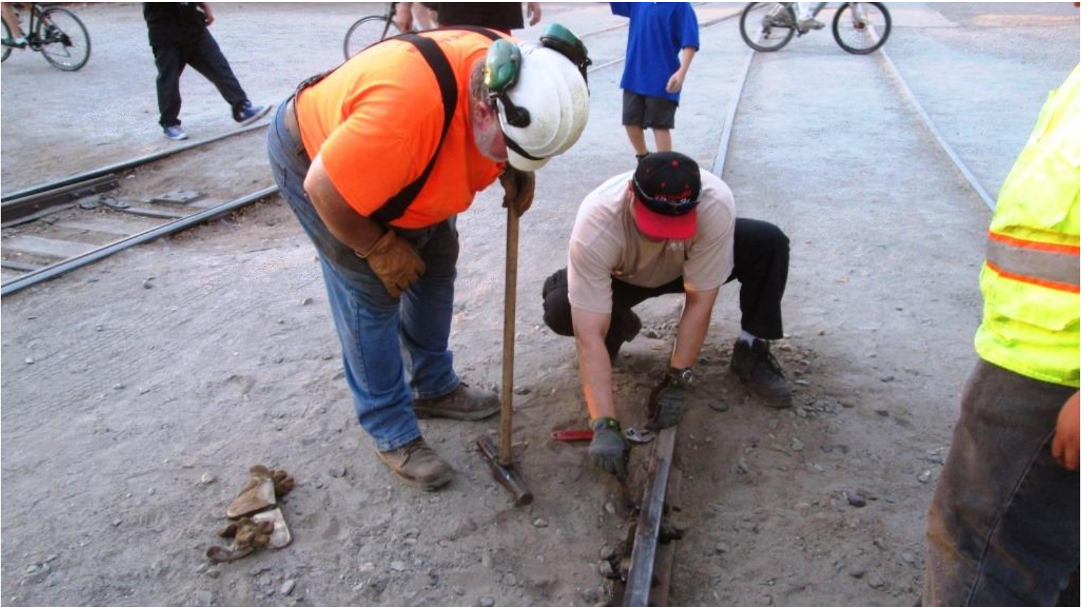
Frank and Jose prepare to re-spike the joint while trying to avoid being trampled-on by pokey-people
