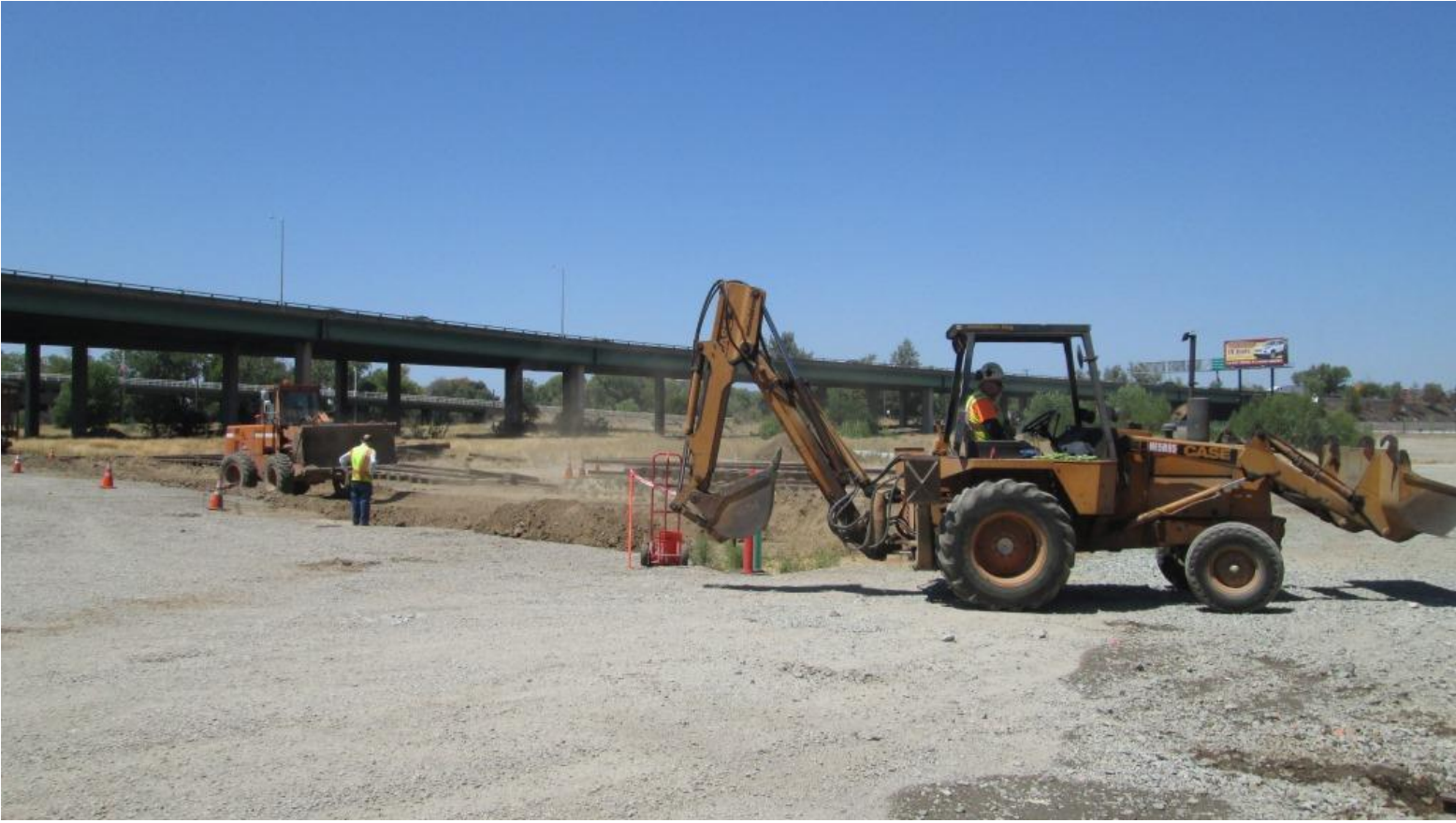
Joe in the loader and Mike F. in the back-hoe take care of the final details
