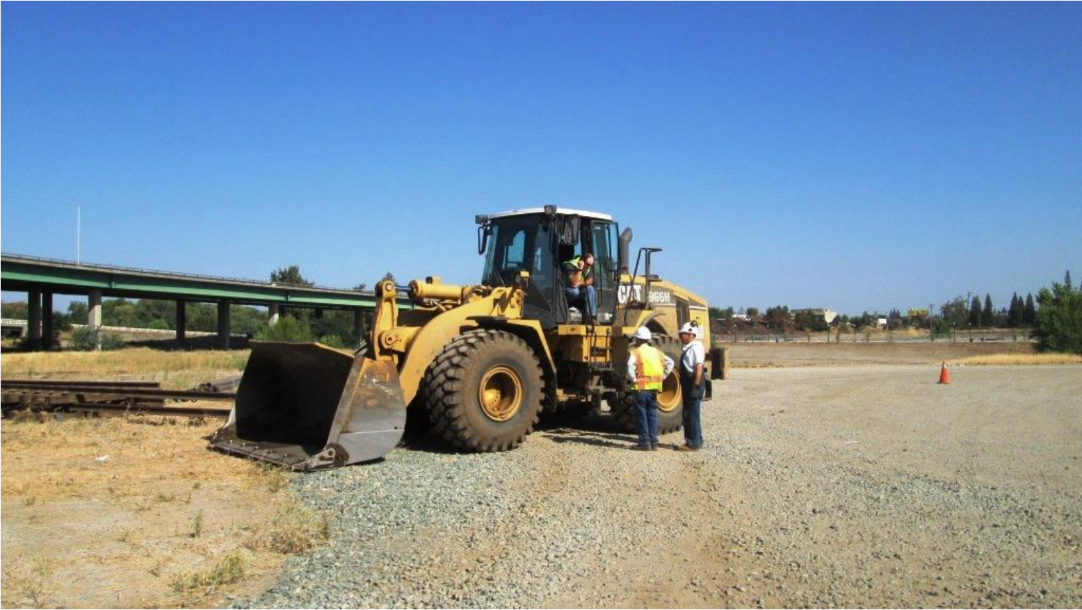
Harry and Clem discuss logistics with the operator of the “big-Cat” from ERM
