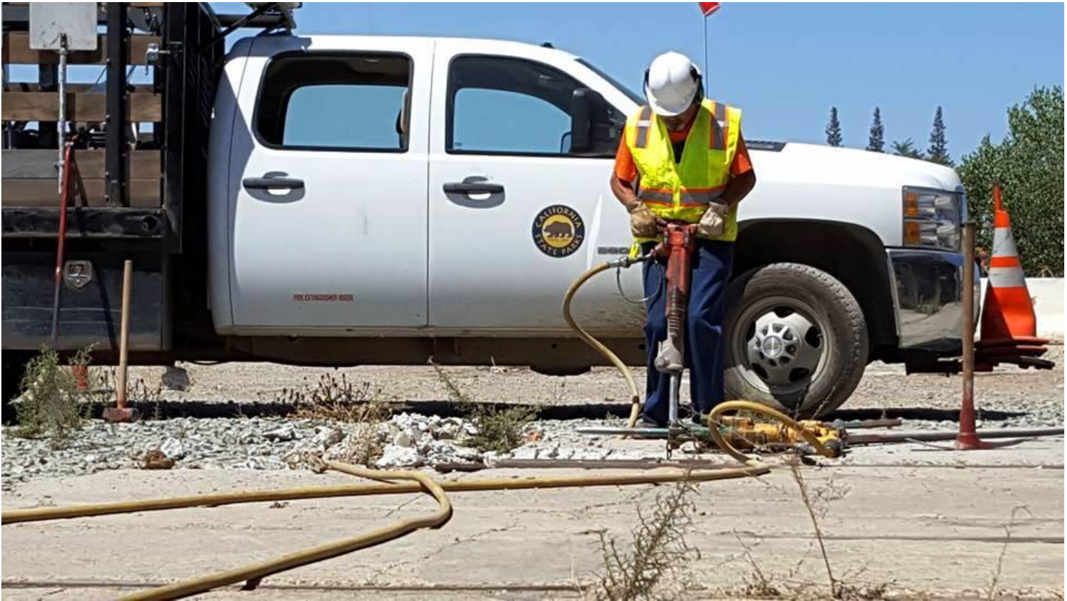
Ed K. takes on the concrete of the north Firing Line track
