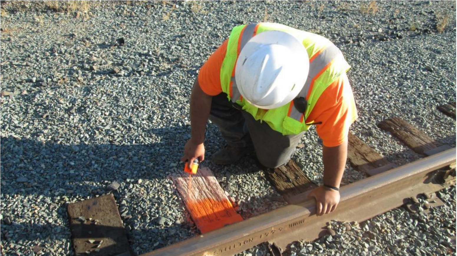
Anthony marks the east approach to the UP Main crossing signal circuit
