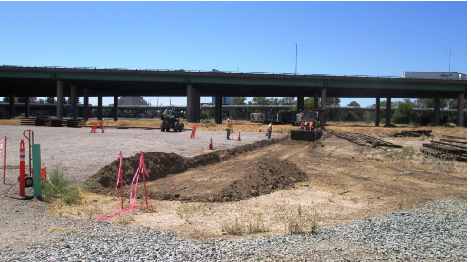
And there it is. The graded roadbed ready for track
