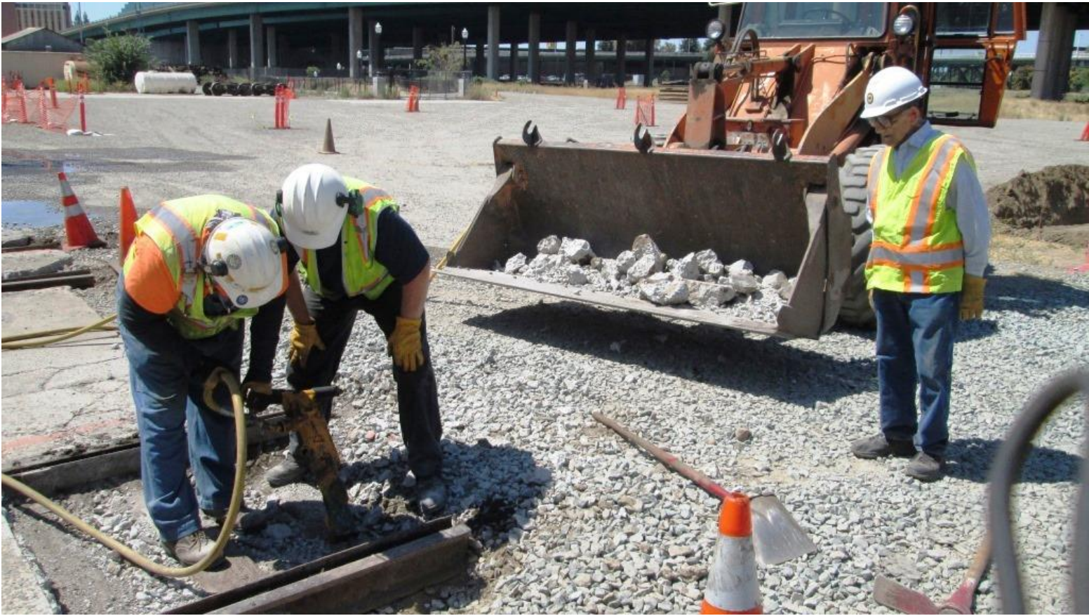
Oops! I think we're stuck. Mike F. and Ed M. work to free the jack-hammer as Harry looks on
