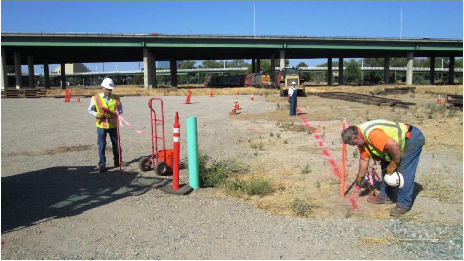
After Harry sighted the center and off-set lines, Frank marked them with marker paint
