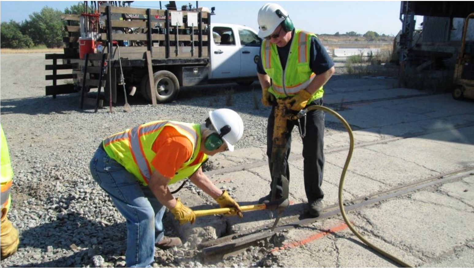
Meanwhile, Ed M. continues to jack-hammer as Mike W. clears away the rubble
