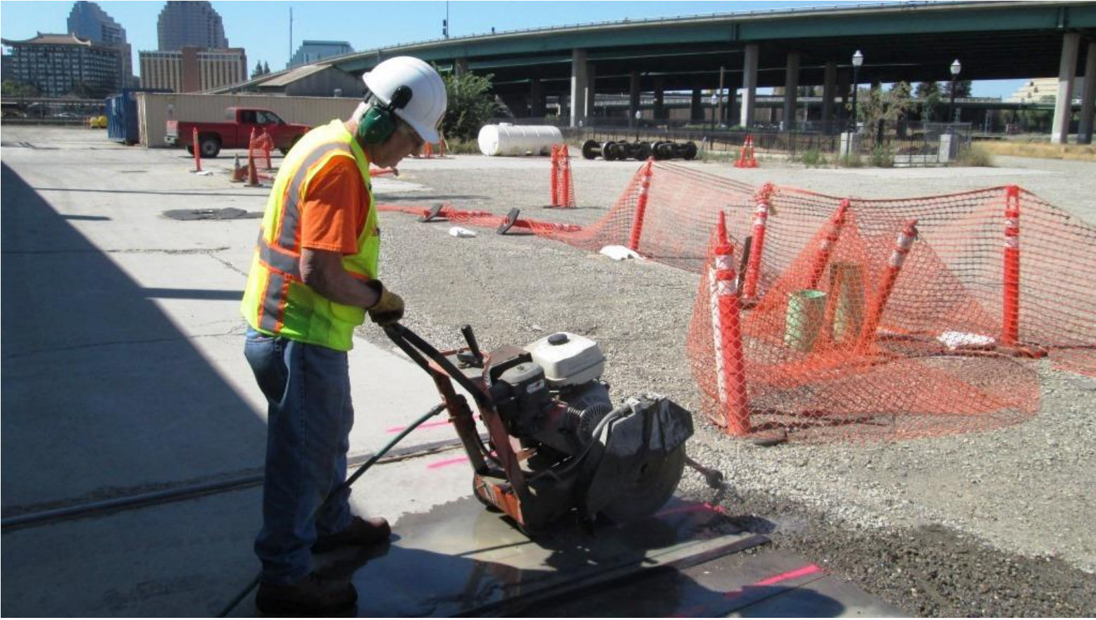
Mike W. takes the helm of the concrete saw
